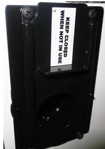
Lift up to open the port to run cables out. -Typical View
